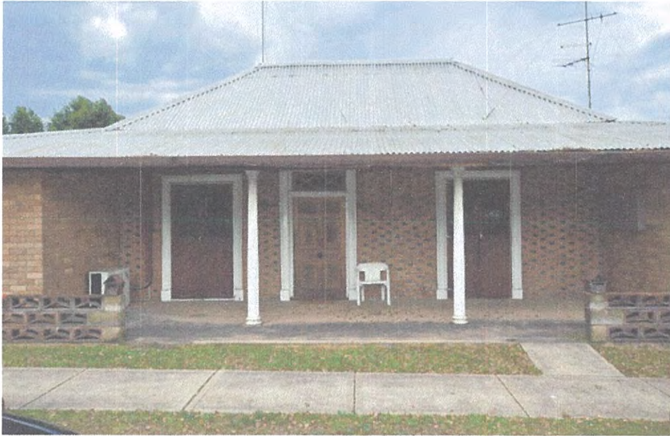
Views of 77 Main Street from street frontage
